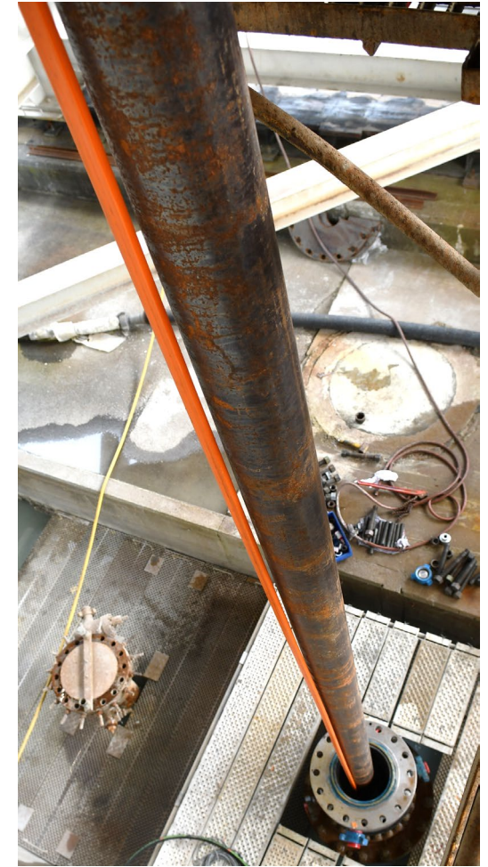
Running 6 5/8" tubing + flatpack into P&A well U8
