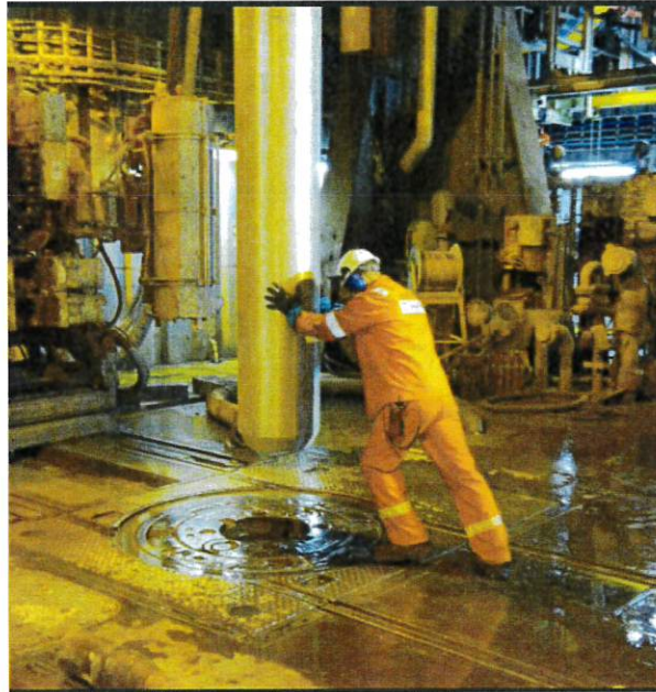
Figure 8 Installing a Bismuth alloy plug on Valhall DP
