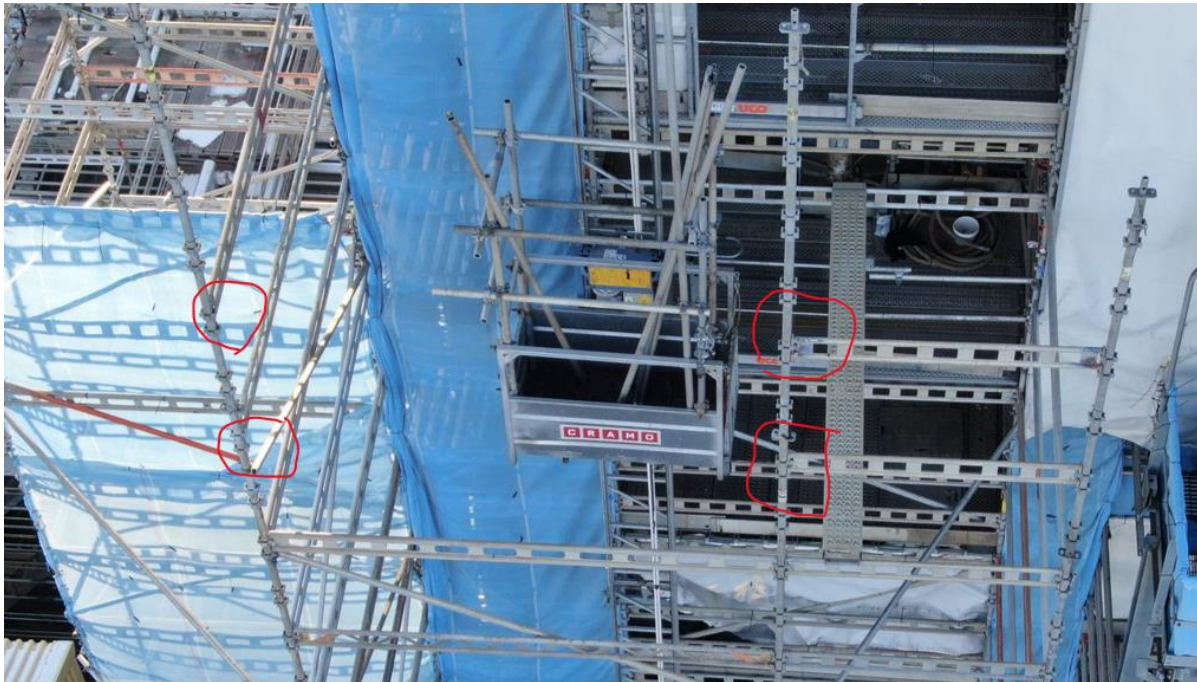
Figure 11. Ledger attachment site marked by red circle.
