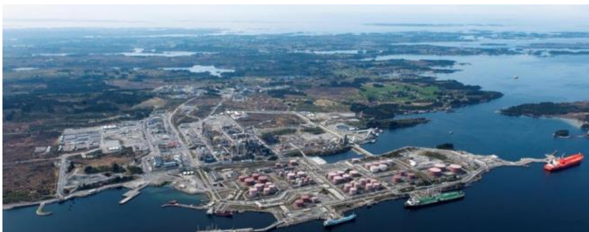
Figure 1. Panoramic view of the Mongstad plant. (Source: Equinor.com)
