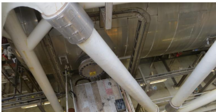
Figure 2 The inlet separator with manway cover closed. Photo PSA
