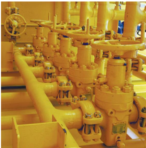
Figur 8-10 Graylock clampforbindelse (ref. Graylock brosjyre 05/08)
