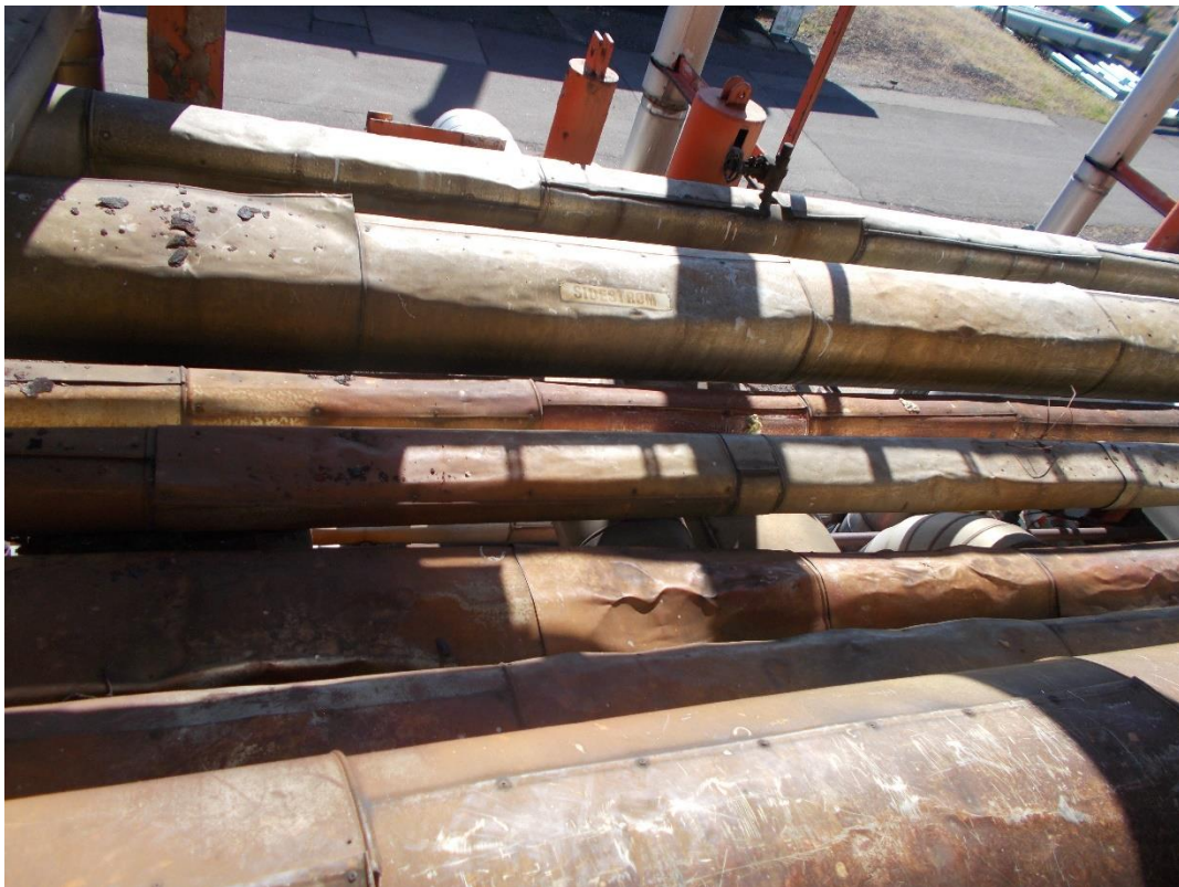
Figure 10: Condition of insulation jackets on surrounding pipes close to the leak.
