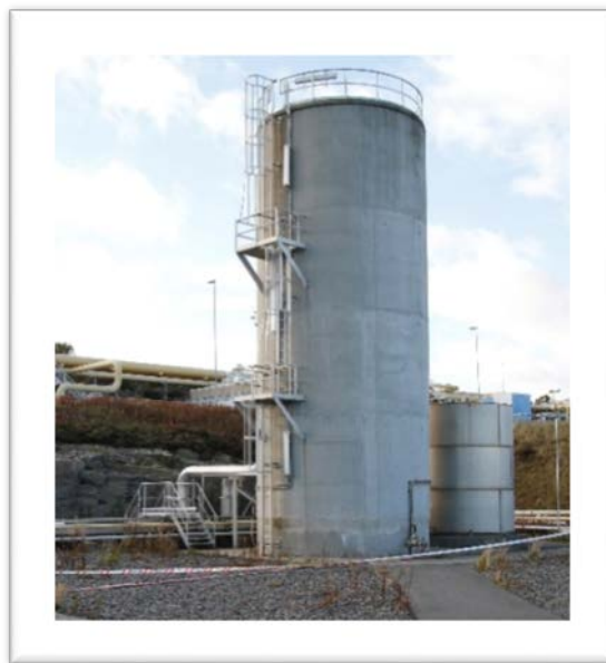
Fig 2. H 2 S reactor (source: police)
