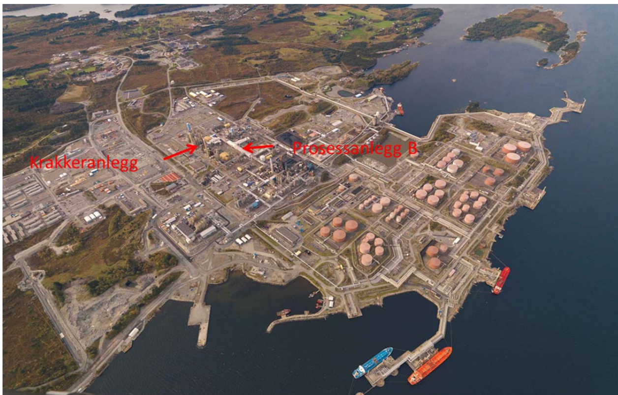
Aerial view of the Mongstad refinery. The leak occurred in the cracker (red arrow). Key: Cracker; Process plant B.
