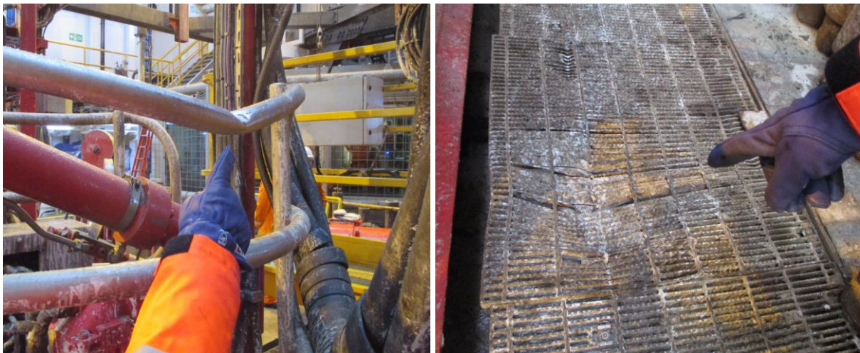
Figure 16 Damaged railing and deck grating.
