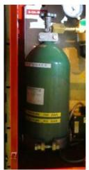
Figure 4: A 3.4 litre nitrogen gas cylinder. (Source: Safety Alert/Equinor)
