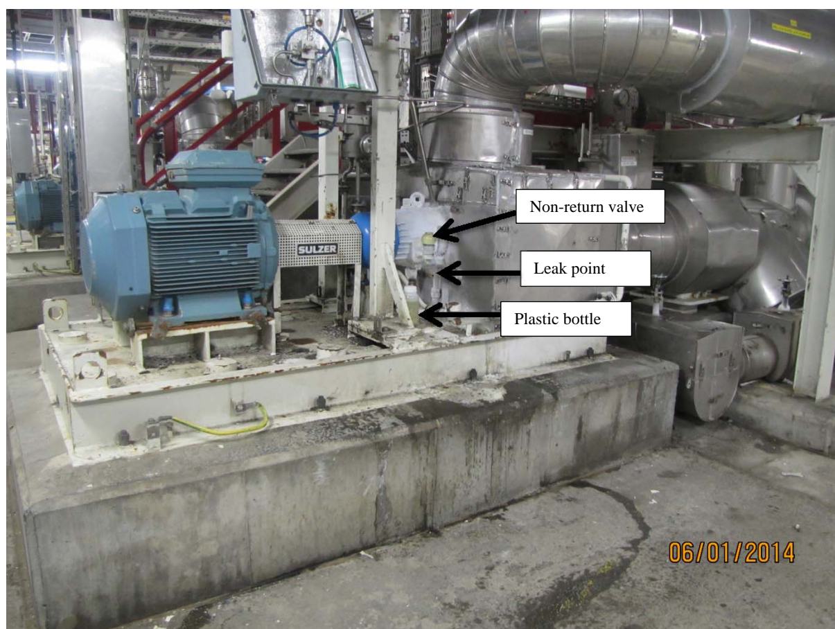
Illustration 3. The leak site.
