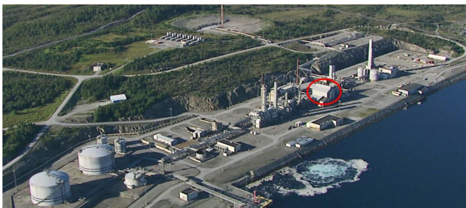
Figure 1 The TBO plant (source: Equinor).
