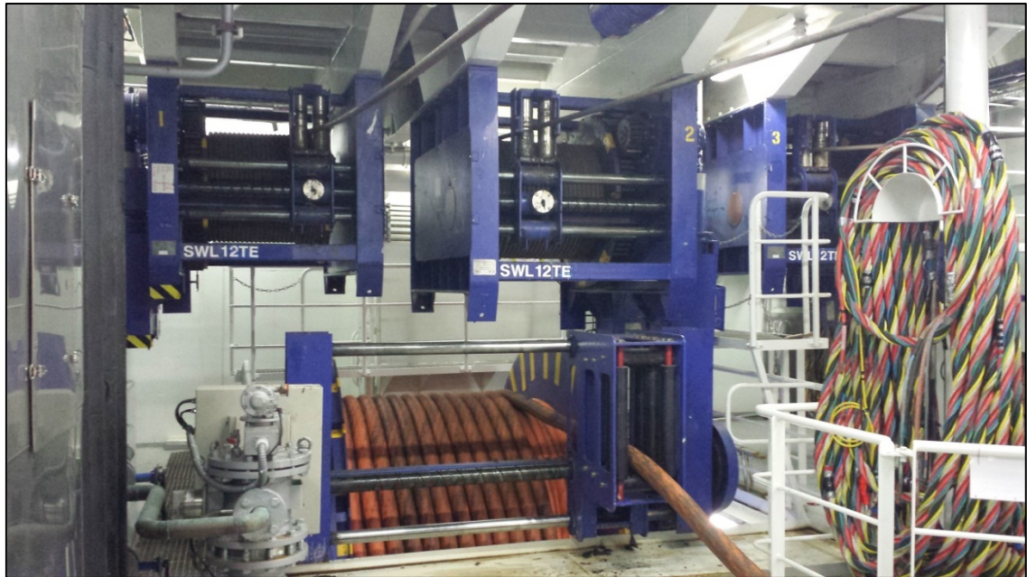
Figure 0-4: PICTURE 1 - 3 x wire winches and 1 x umbilical winch (port side)
