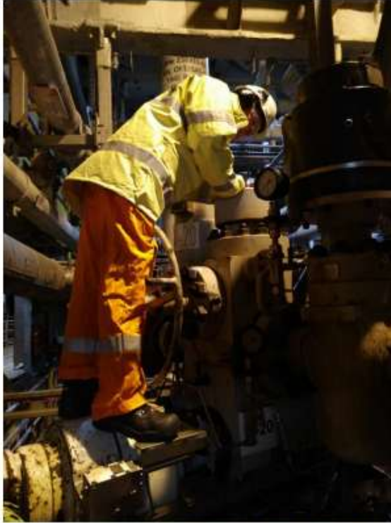
Figure 6 The process technician's working position. Havtil reconstruction.
