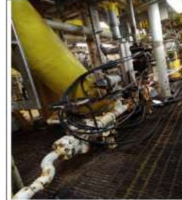
Figure 7 Hose to closed disposal system
