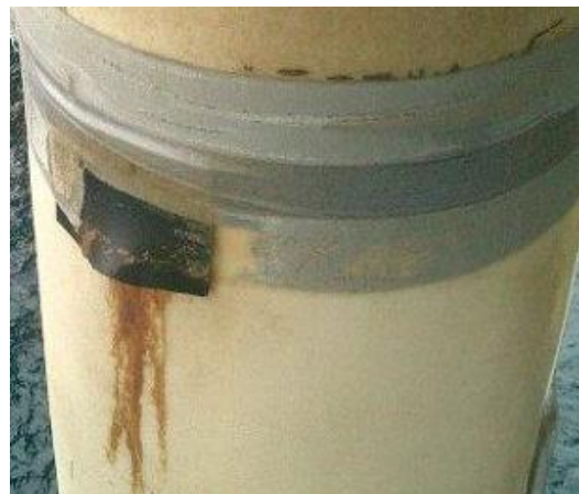
Figure 5-3 Less successful annulus vent backup system
