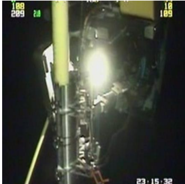
Figure 5-12 ROV installable clamp stop oxygen ingress to armour wires (4Subsea)
