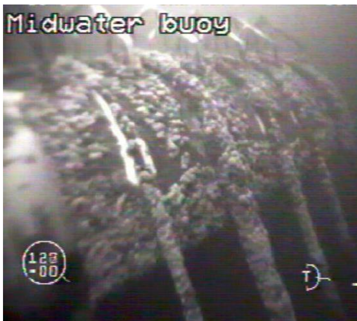
Figure 4-11 Mid-water arch with marine growth (pipe dynamics seen as white areas) (Talisman)
