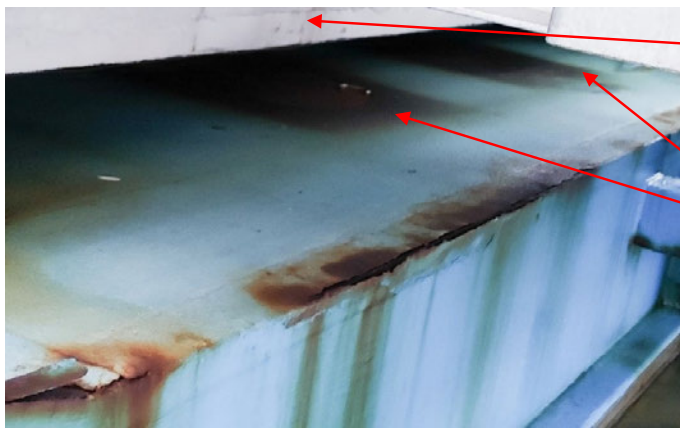
Figure 18 Top of the roof of the high voltage room after the fire (Source: Havtil)
