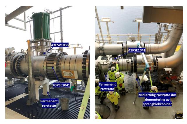
Photos 1 and 2: Taken at the incident site while disassembling the rupture disc on 11 April 2019 (PSA).
