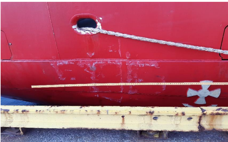
Photo: Dented deck plate.
