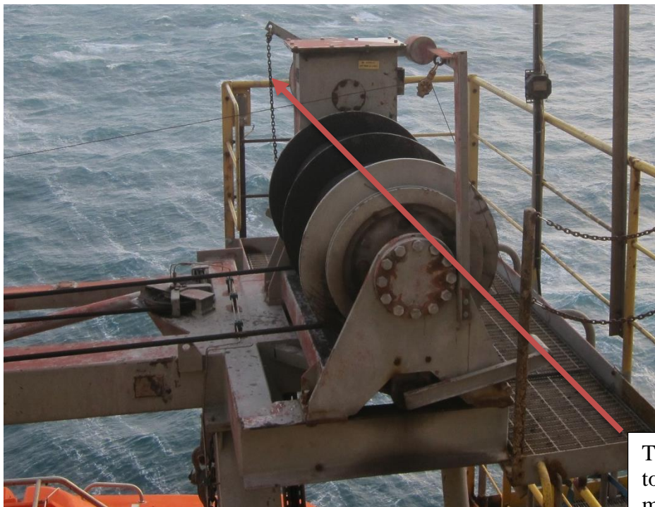
Figure 3: Overview of the winch system on the corresponding port-side davit.
