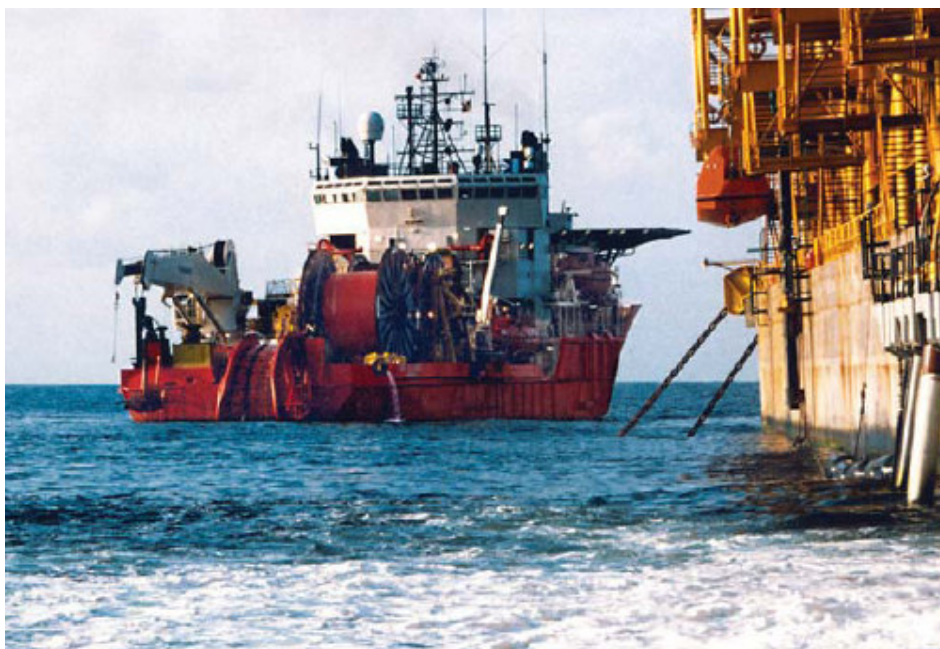
Figure 3-5: Flexible pipe installation (Technip)
