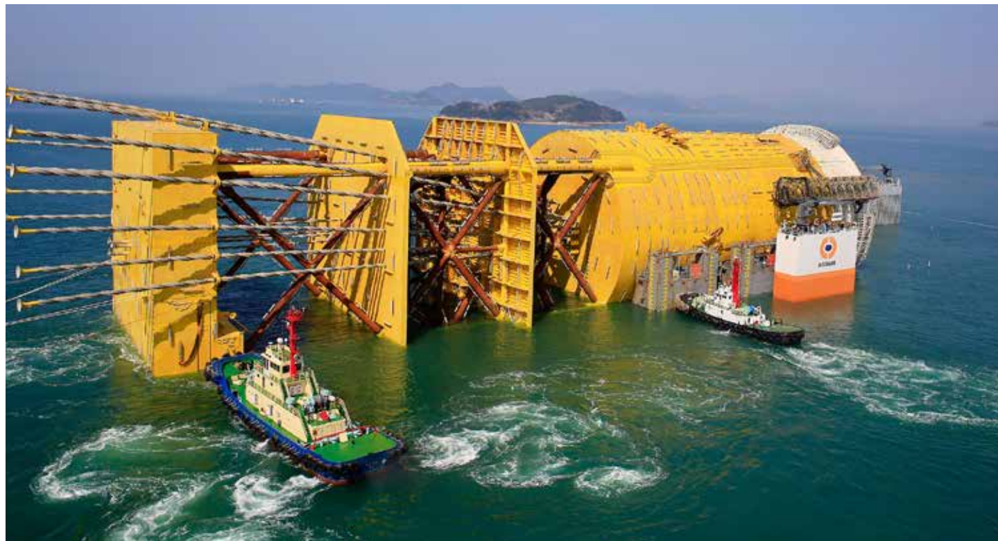
Aasta Hansteen is one of the newest fields to come on stream off Norway. It has been developed with a Spar platform, seen here being transported from the yard in South Korea to Norway. (Photo: Boskalis/Equinor)
