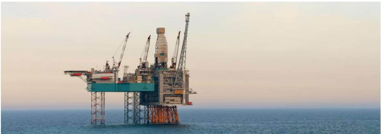
Figure 9-5 The Rowan Viking jack-up drilling rig is positioned immediately next to the bottom-fixed Edvard Grieg Platform /51/
