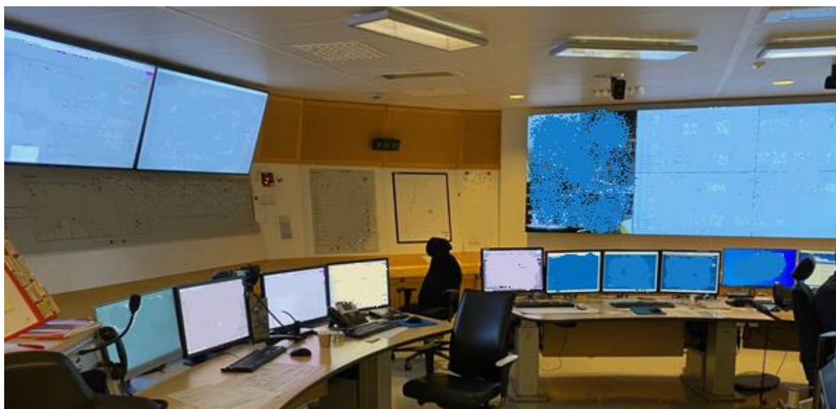
Figure 9 The CCR with big screens, fire, gas and ESD overviews and operator monitors. Photograph: Equinor.
