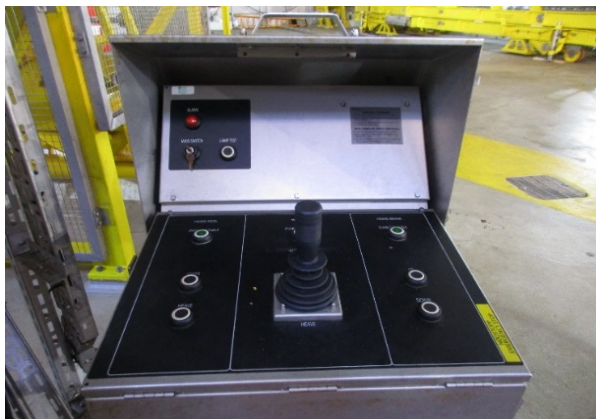
Photograph 7: Control panel of the work winch (tag 33MK003). (Source: PSA)
