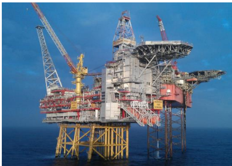
Figure 2: The Gudrun platform. Source: Equinor
