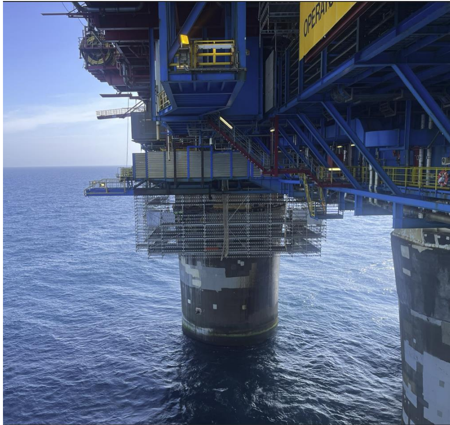
Ringstillas for rehabilitering
