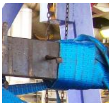
Photograph 9 Deformed deck grating fastener where the grating came loose.
