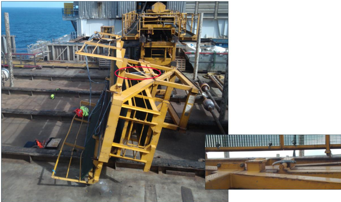
Figure 5 - The structure where the wire rope sling became snagged. From Equinor’s presentation of the incident.
