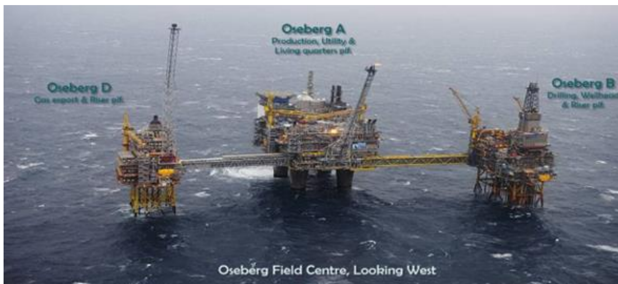
Figure 1 – The Oseberg field centre, with Oseberg B to the right.
