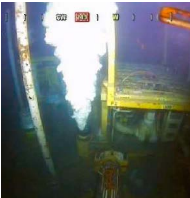
Figure 1 - Photograph of the gas leak (Source: Statoil)
