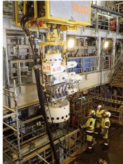
Gudrun – overhead crane setup
