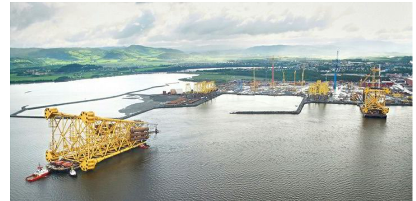
Jacket fabrication, Aker yard in Verdal (Norway)
