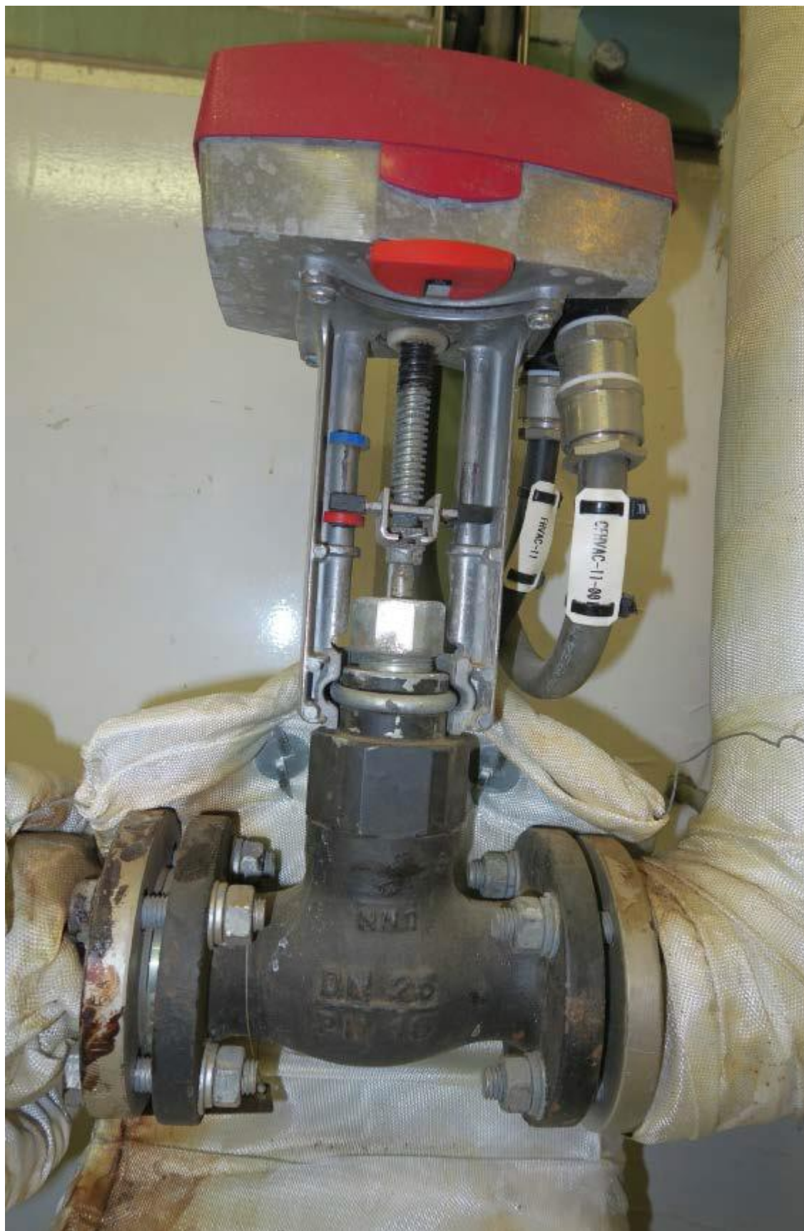
Figure 2 TAC-type steam valve, model number VGS211F-25-10, with Schneider M800 actuator (source: TKPJ).
