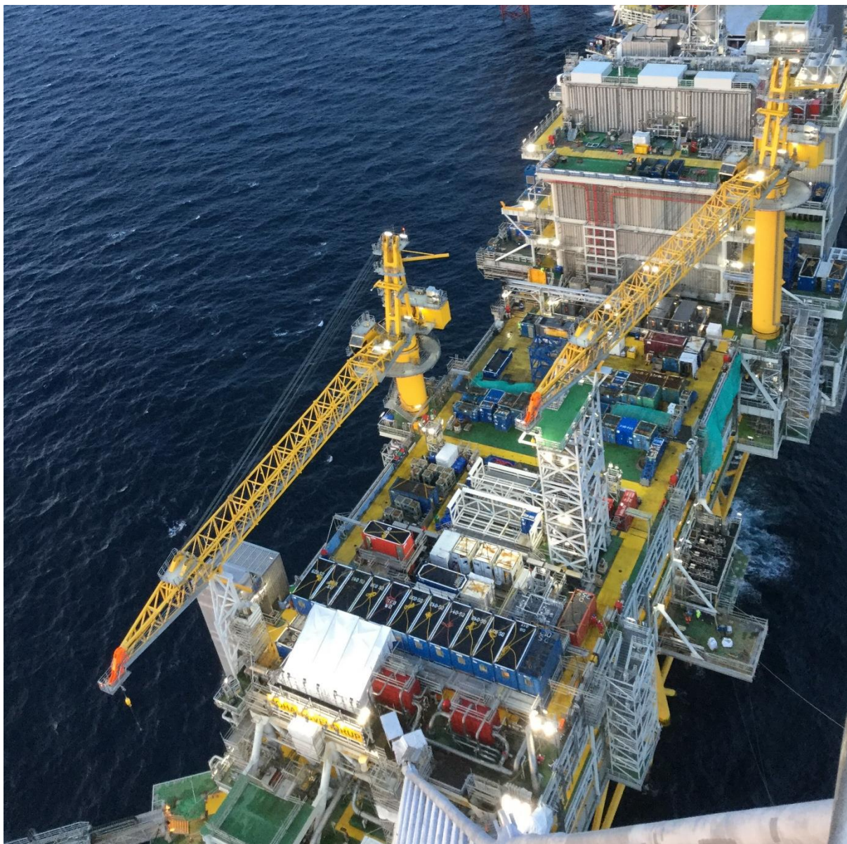
Photo 2 has been received from Equinor and shows the RP.
