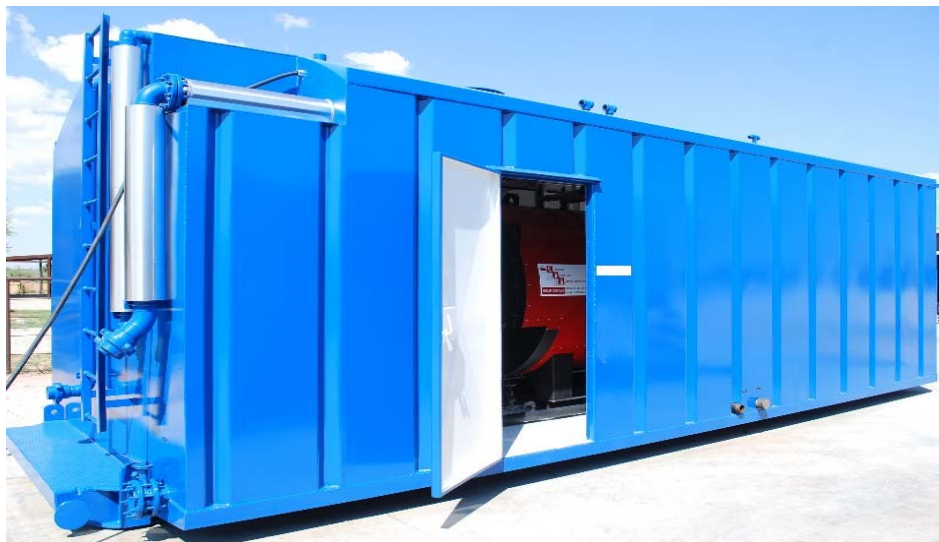
Figur 8-28 Damp enhet i kontainer for Sakhalin (ref. Hurst Boiler)
