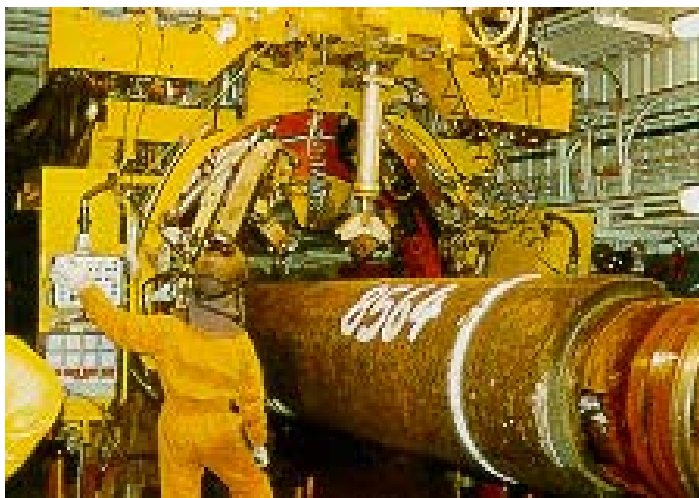
Figure 4. Saturnax welding system (LB 200), and detail of welding heads.
