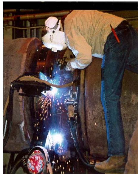
Figure 3. Installation of line-up clamp (SOLITAIRE) and the Phoenix welding system (Soiltaire).
