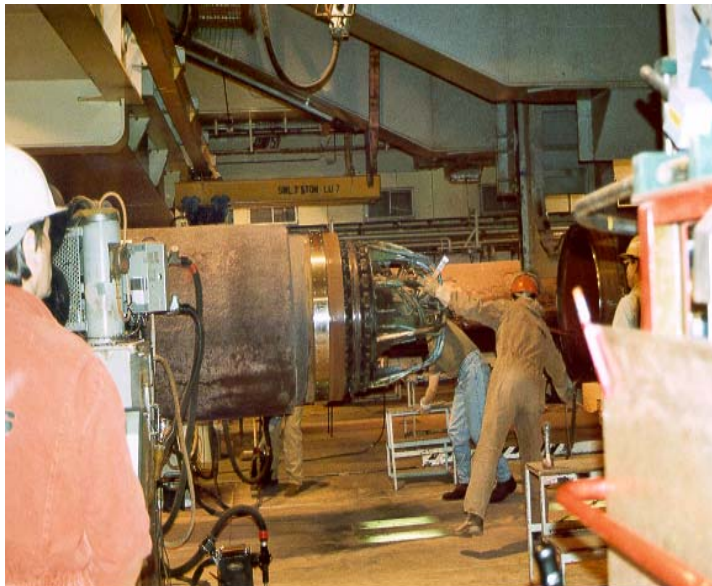
Figure 3. Installation of line-up clamp (SOLITAIRE) and the Phoenix welding system (Soiltaire).
