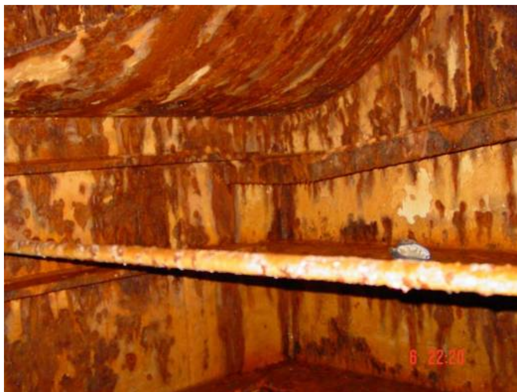
Figure 3-2-3 General Corrosion inside ballast tank (DNV photo).
