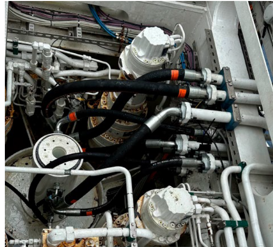
Photo 6: Swivel with temporary hydraulic hoses (Source: Equinor/Island Offshore)
