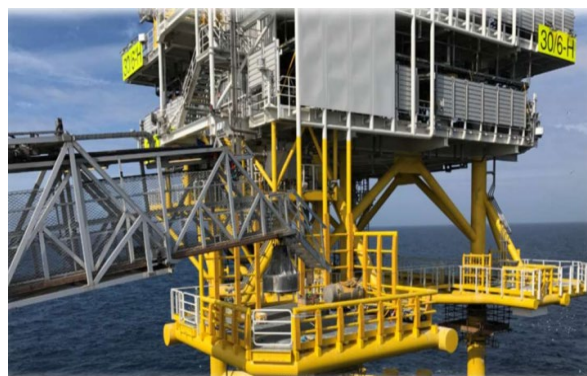
Photo 3: Eastern landing area with W2W system in cone mode. (Source: Equinor)
