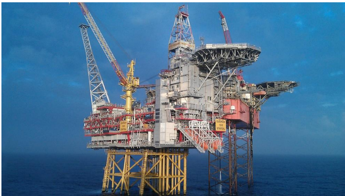
Photograph 1: The Gudrun facility. (Source: www.statoil.com )
