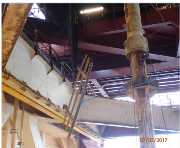
Figure 13 The railing was broken off and fell towards the BOP deck, where it landed in the safety net.
