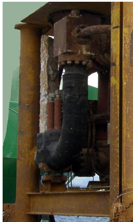
Figure 7.3 Use of rubber coating on piping
