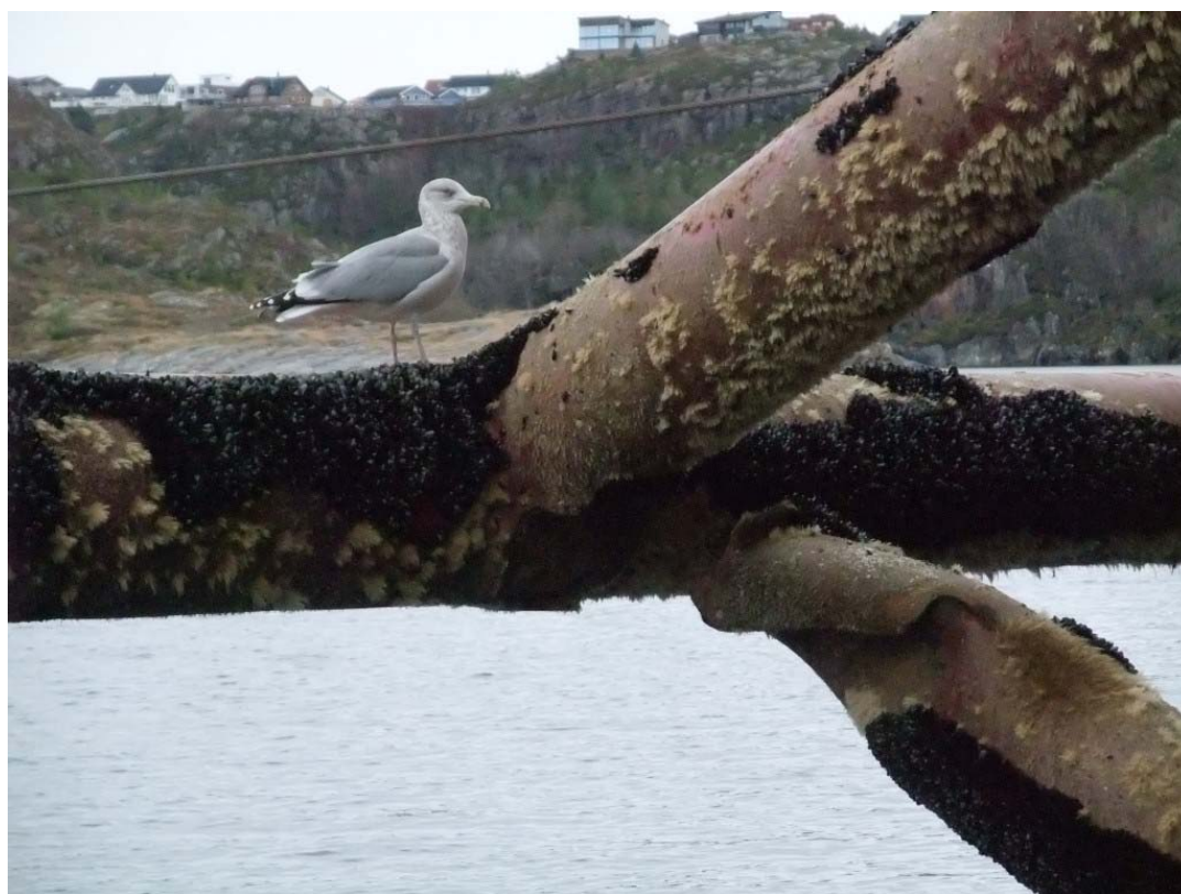
Figure 28: The bolster on the forward port side. Anchor 1 has hit the brace under the bolster bar. Note that the lower brace has been disconnected completely and shifted about one diameter aft (to the right in the photo), and is thereby attached only at a point on the side of tank 3A starboard. The damage is not the outcome of a sudden fracture, but has big deformations from action over a long time. The bolster at anchor 8 (A in Figure 27) has probably suffered similar damage on the evening of 6 November 2012 (all the anchors have damaged bolsters). The photograph was taken in Kristiansund on 13 November 2012 by the PSA.
