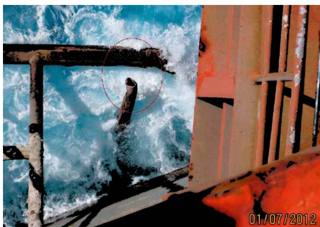
Figure 46: Brace cut off on the bolster on West Hercules 1 July 2012. Photograph: Seadrill [128].
