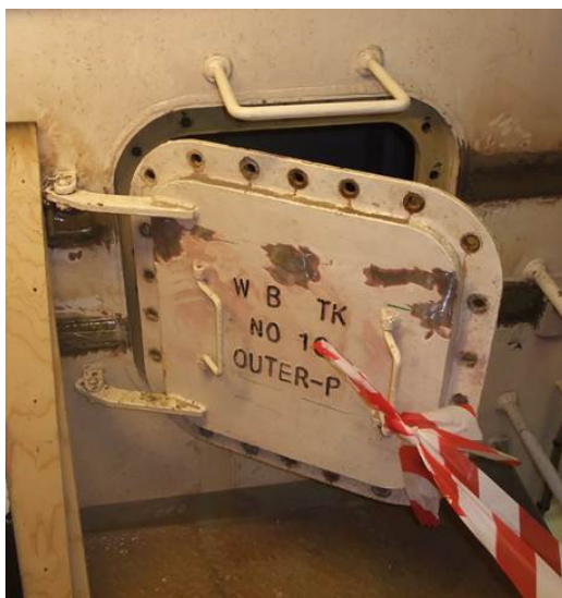
Figure 8: Hatch from the central column to ballast tank WB TK NO 10 OUTER-P. Marks from the reinforcement temporarily welded on during 7 November 2012 are visible where the paint has gone. Seal and bolts are removed. Photograph taken by the PSA in Kristiansund on 12 November 2012
