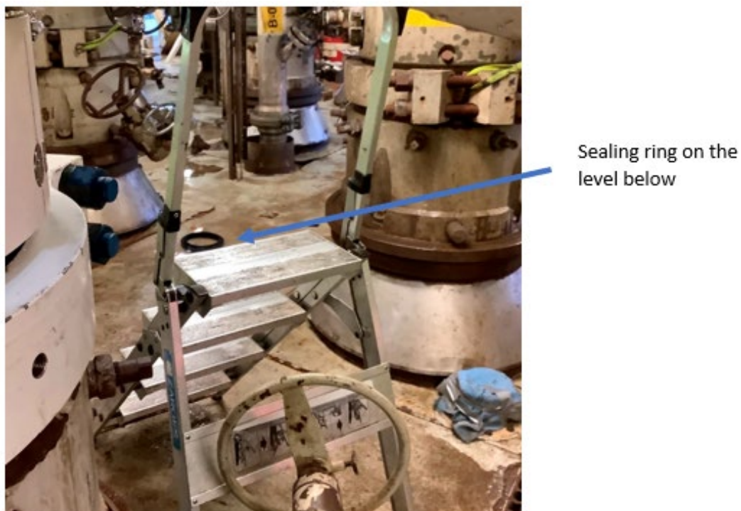
Figure 13 Photo of the sealing ring which hit the person on the deck below the area where the incident occurred. (Source: Equinor)
