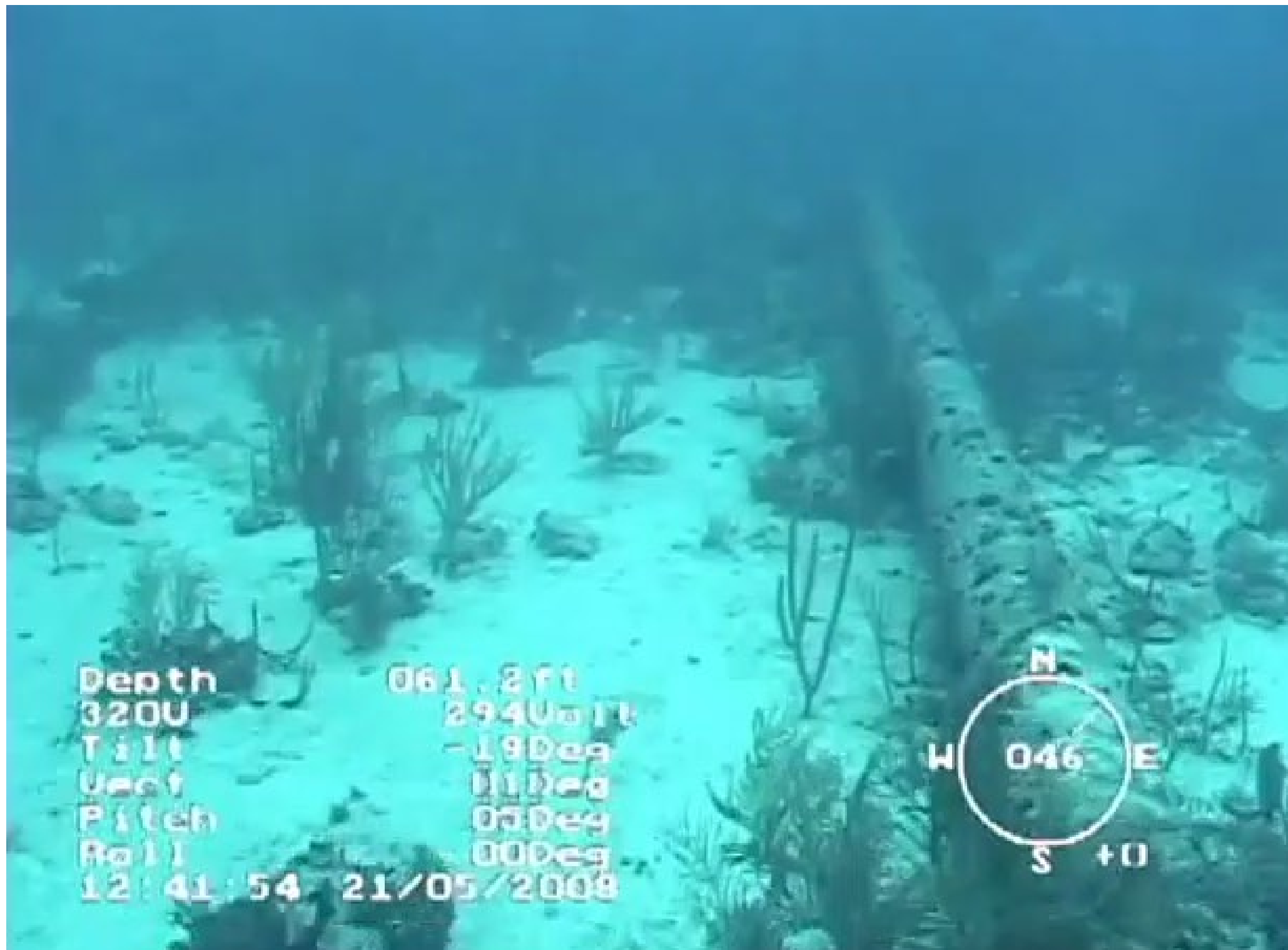
Pipeline inspection with a Remotely Operated Vehicle
